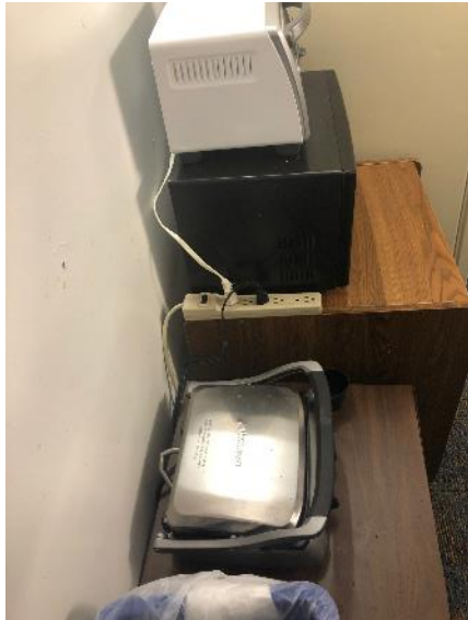
Evidence of Inadequate Power Capacity / Wiring Integrity
