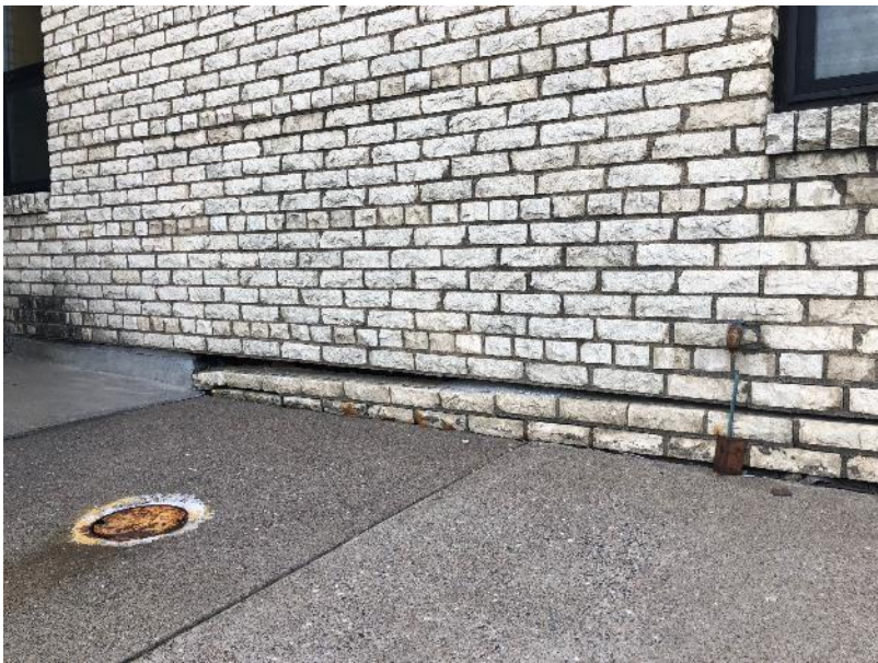
Evidence of Exterior Wall Failure
