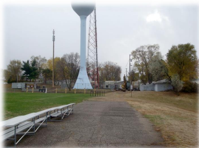
The path to the Hilltop community is not paved and lacks lighting currently.
