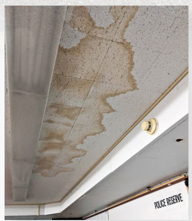
Water damage from roof and wall leakage is prolific throughout the building, in some cases leading to visible mold growth.
